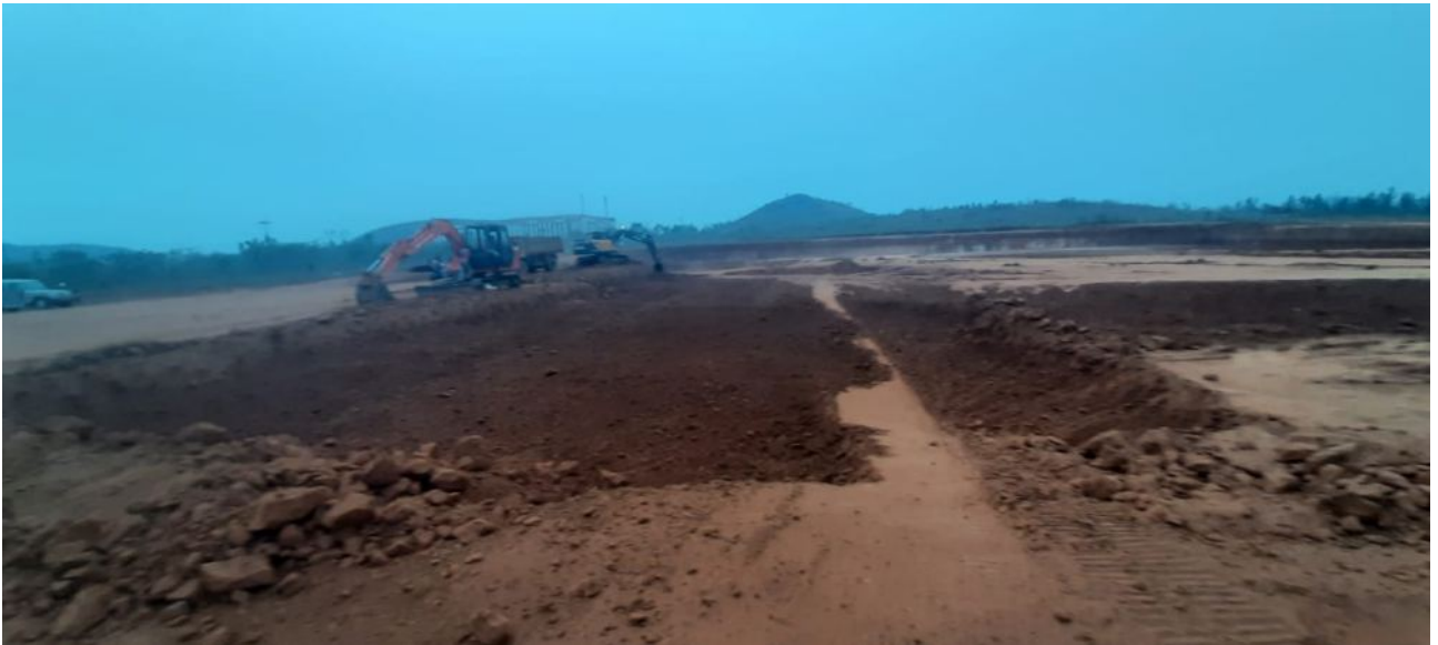
The preparation work of playground is in progress at CUO campus
