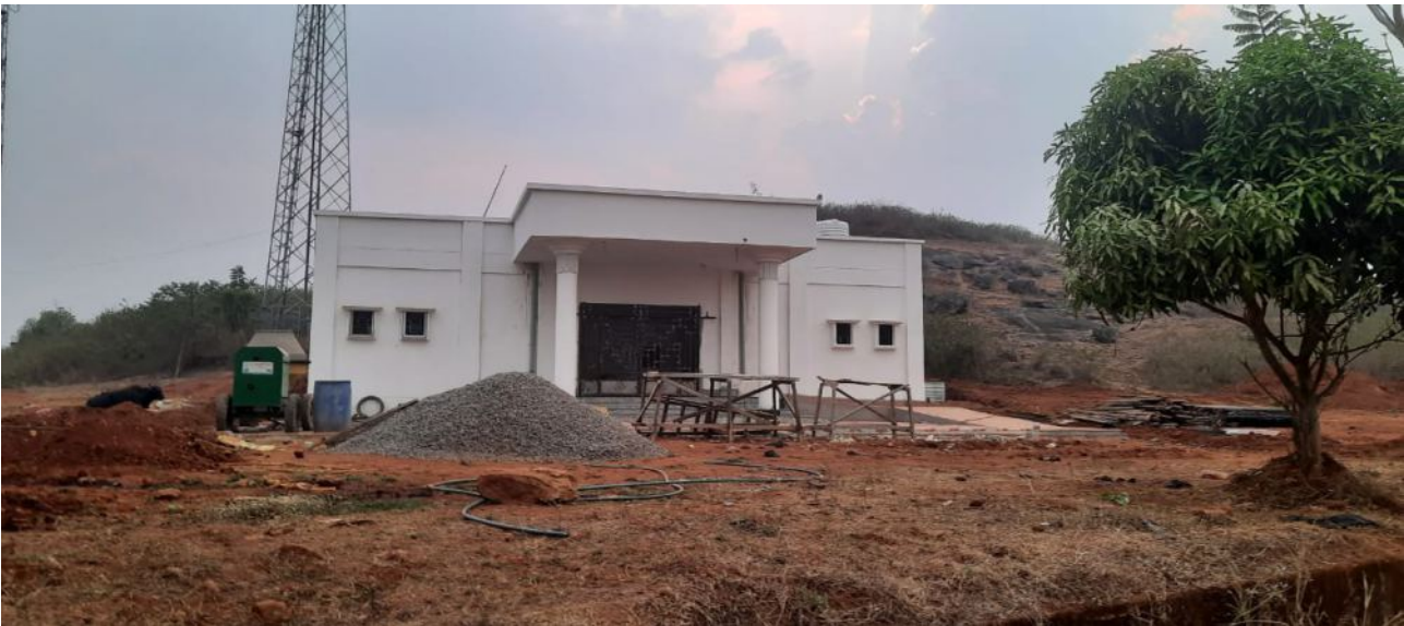
The construction work is in verge of completin
