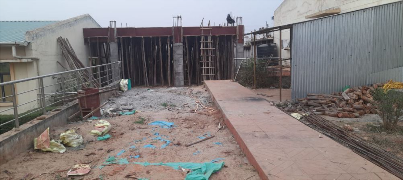
The construction work of Extension of Library is in progress
