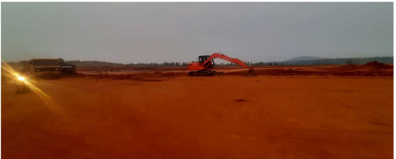
The preparation work of playground is in progress at CUO campus
