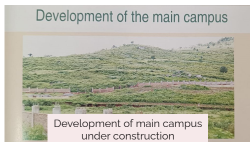
CUO boundary wall on the main campus site
