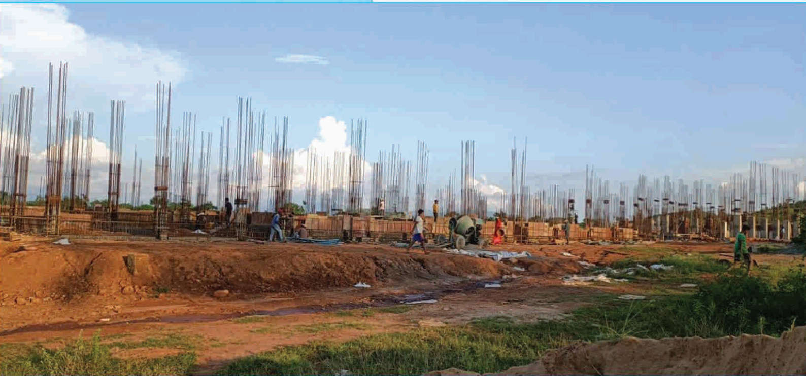
Construction of Academic Building at CUO campus in progress
