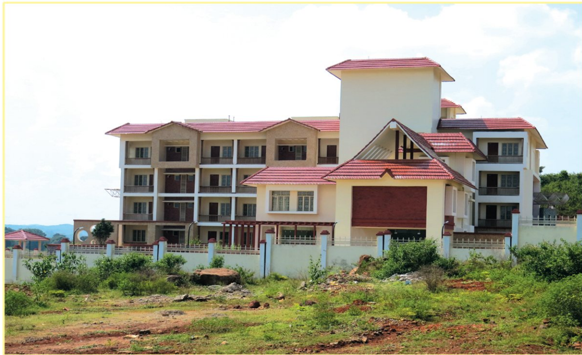
Guest house at CUO Permanent Campus, Sunabedha
