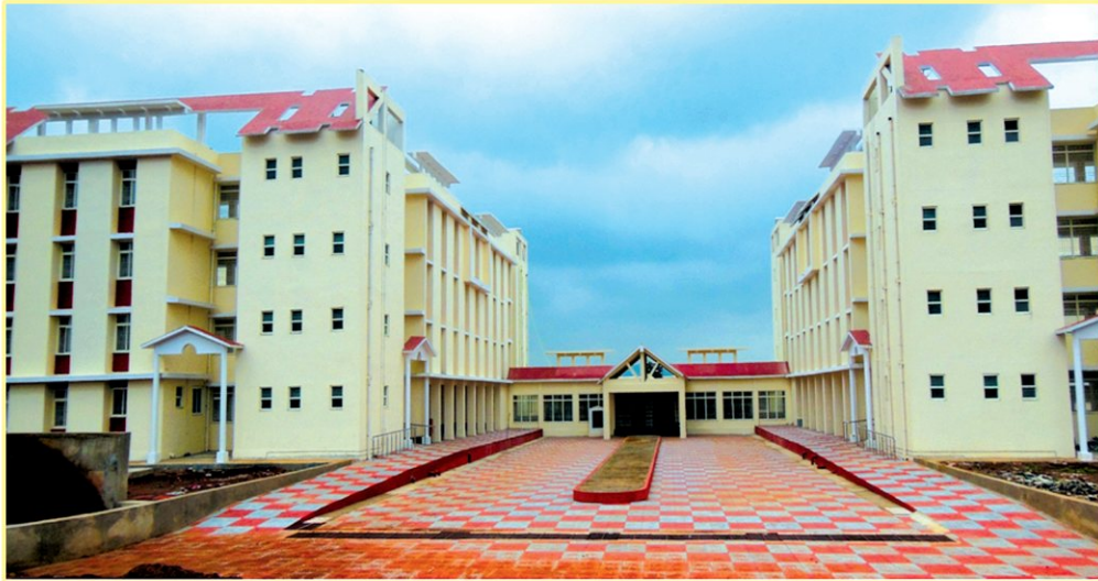
Boys' Hostel at CUO permanent Campus, Sunabeda will be opened shortly.
