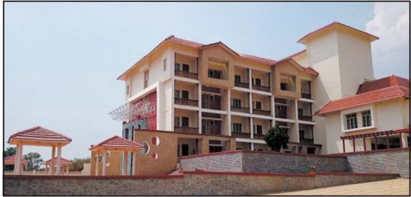
Guest House at the permanent Campus of CUO, Sunabeda.
