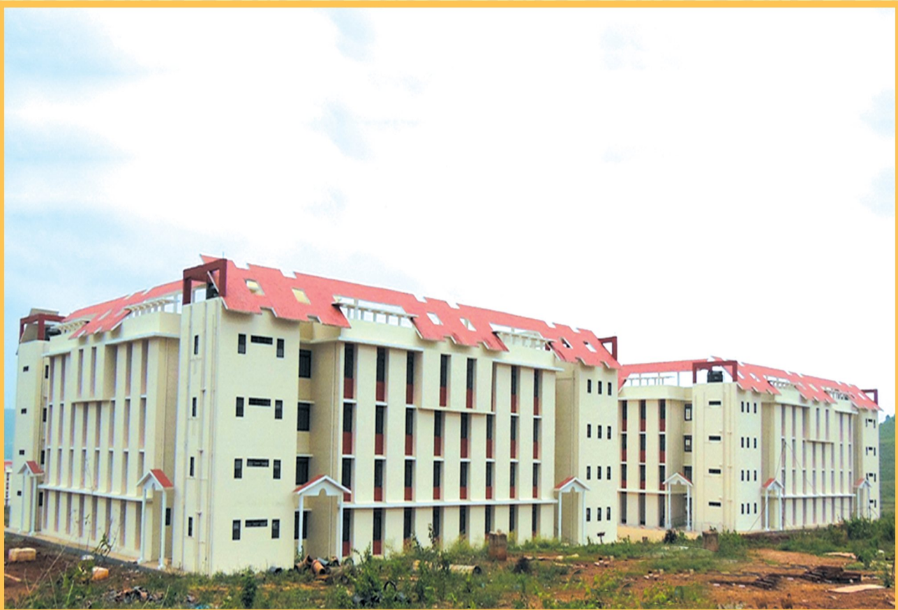
Girls' Hostel at CUO permanent Campus, Sunabeda
