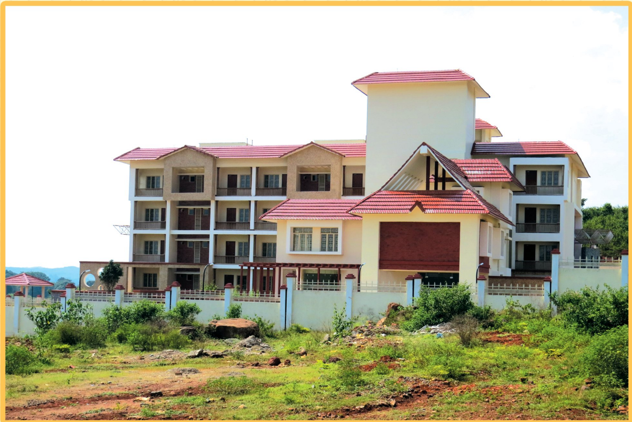
Guest house at CUO Permanent Campus, Sunabedha
