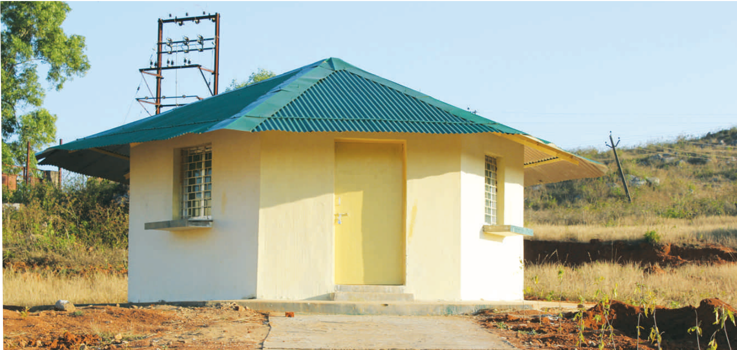
The newly constructed students Canteen inside the Landiguda Campus of Central University of Orissa, Koraput
