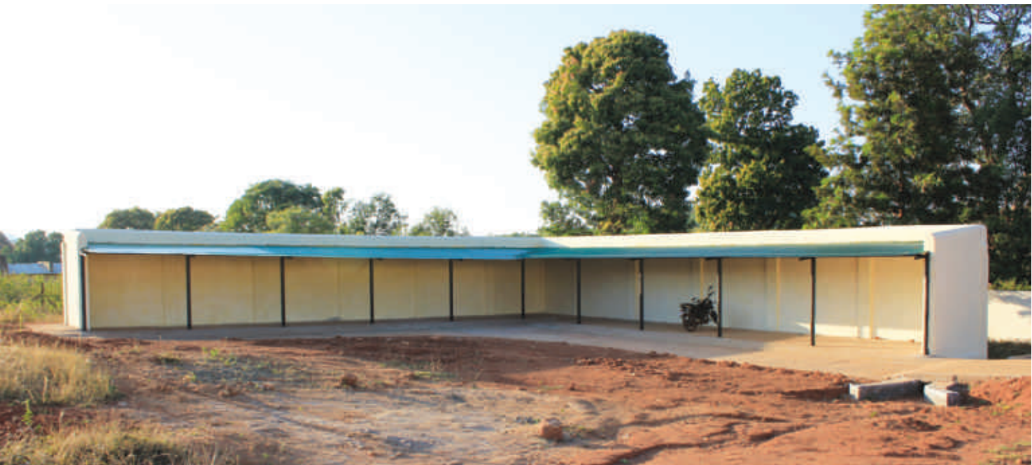
The newly constructed cycle shed at the Landiguda Campus, Central University of Orissa, Koraput
